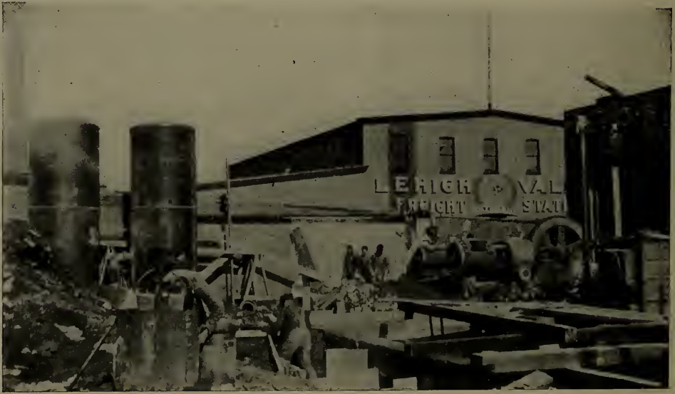
FIG. 9.—Erecting Compressors in Manhattan Power House for the Belmont Tunnels.
